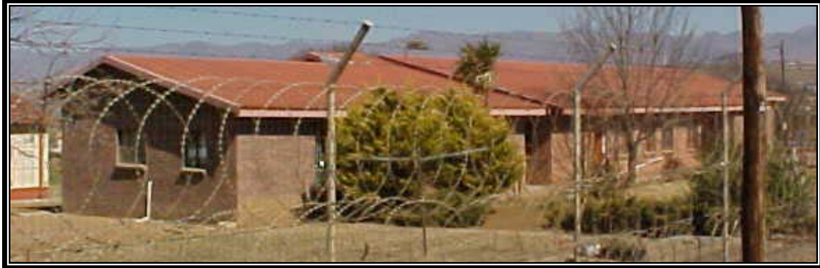
Figure 1: Phuthaditjhaba Clinic Upgrade of Clinic
